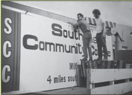
Installing a new road sign on I-80
